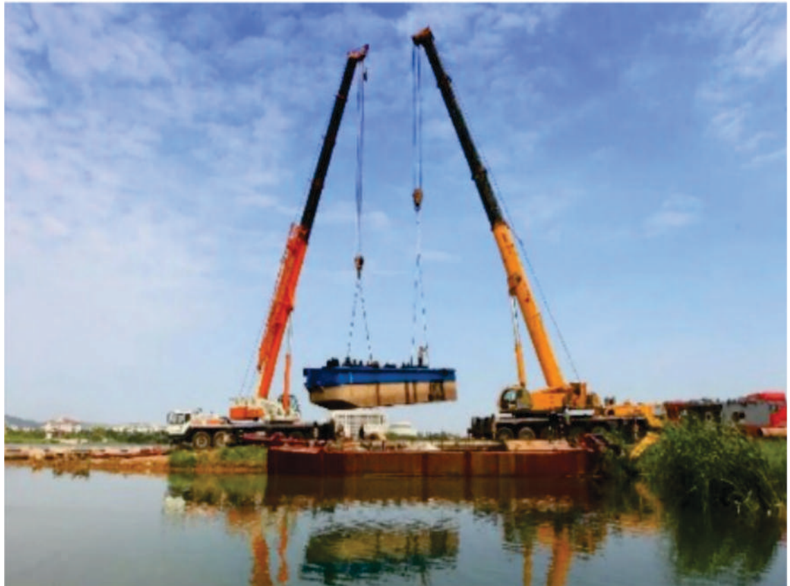
Figure 28: Water operation of large dredger
