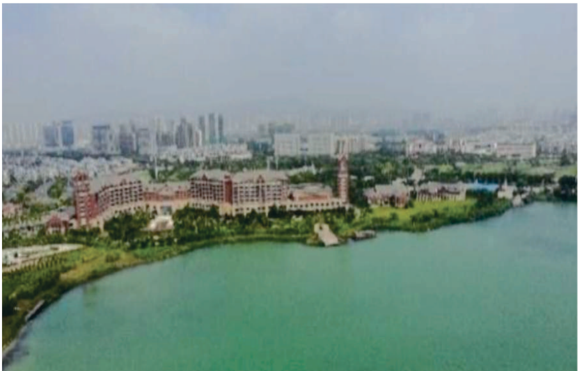
Figure 30: After the treatment of coal mining subsidence area (Lvjin Lake Yuanmeng Island)
