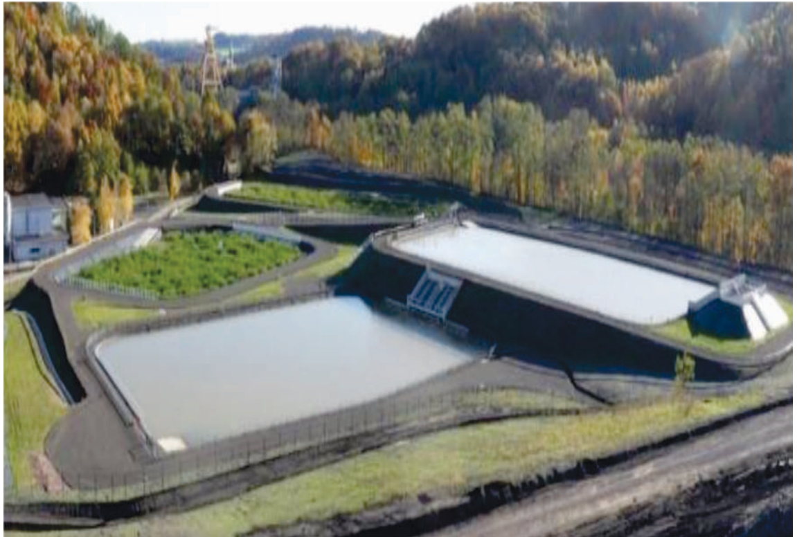
Figure 34: Vouters Coal Mine water treatment station (450 m 3 /h - Pumping + Precipitation of iron and manganese with oxygenation cascade and series of basins)
