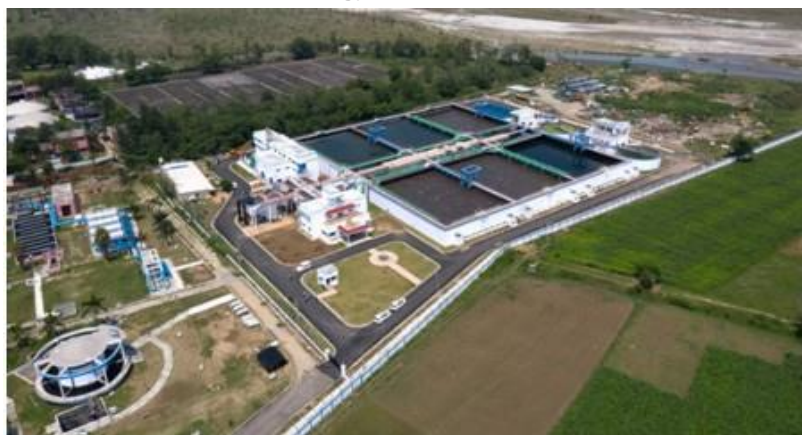
b) 210 MLD Bhingawan STP in Kanpur, Uttar Pradesh
