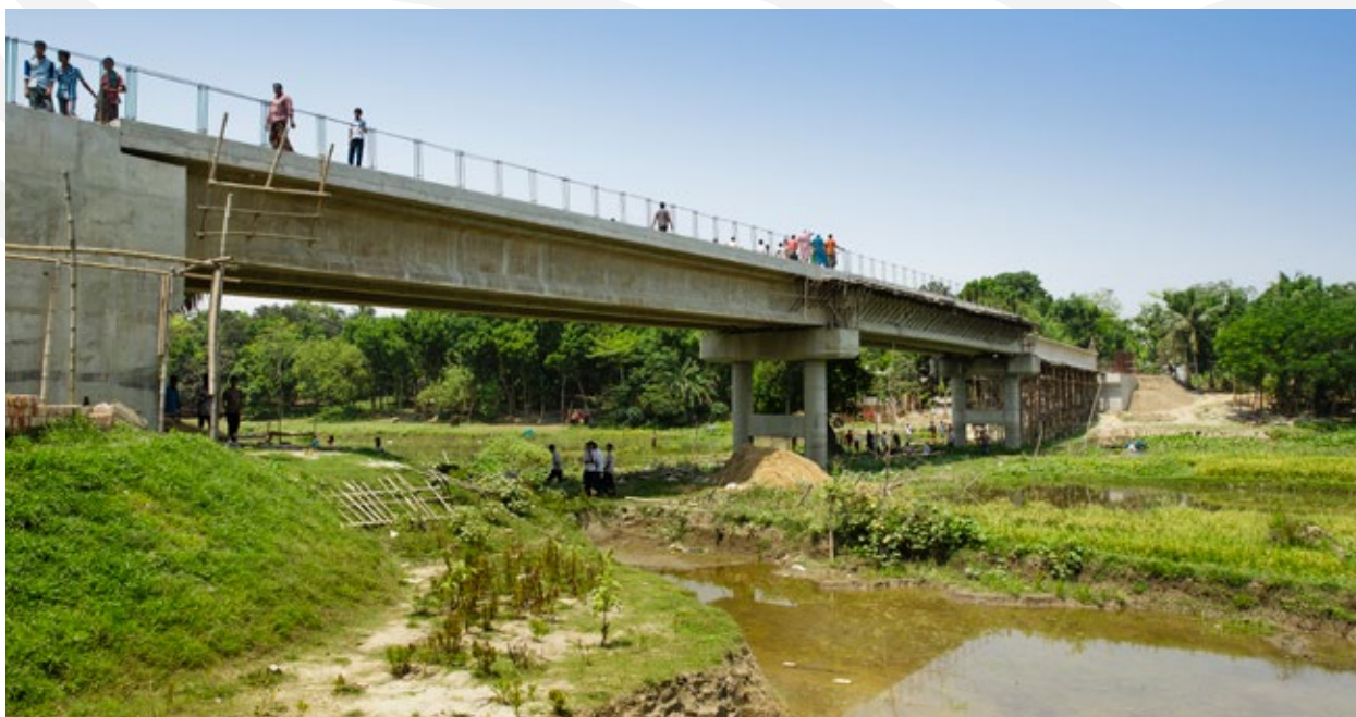
↑ Bridge construction for improved market access (Narikelbari, Bangladesh)
