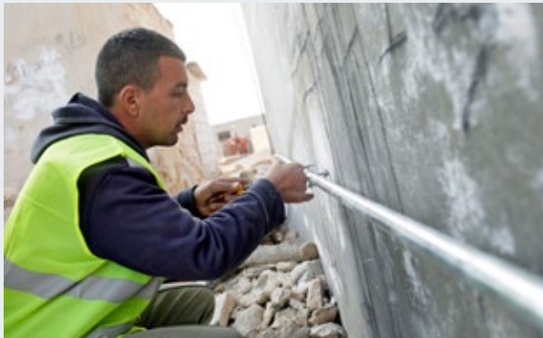
← Installation of drinking water pipes (Mafraq, Jordan)
