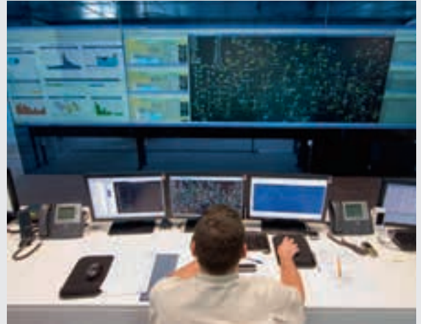
An operations control center in Collblanc, Barcelona, Spain
