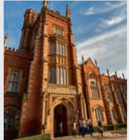
The Lanyon Building, Queen's University
