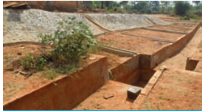
Completed intervention at Ebenebe gully erosion site
