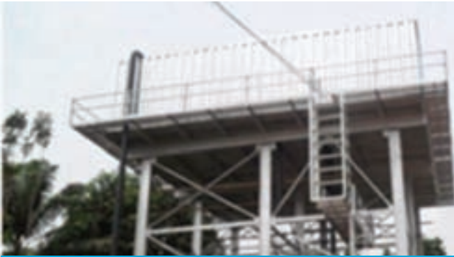
An ongoing Udoka water project in Awka
