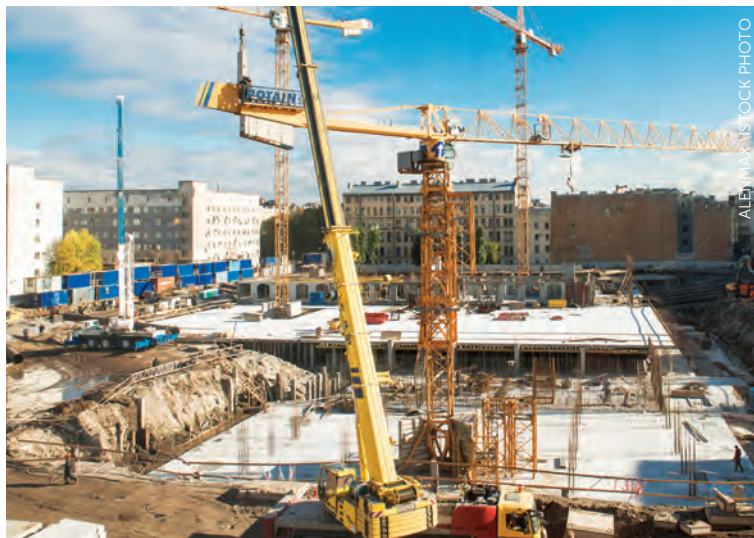
Construction on a residential building in Saint Petersburg, Russia
