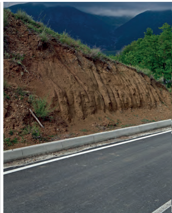
Upgrading roads in Albania with the support of the EBRD, the EU and the EIB
