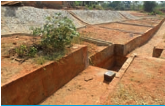
Completed intervention at Ebenebe gully erosion site
