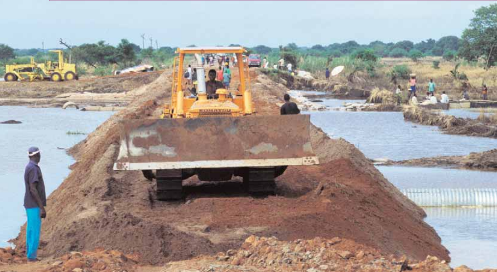
Road repairs in Palmeira, Mozambique
